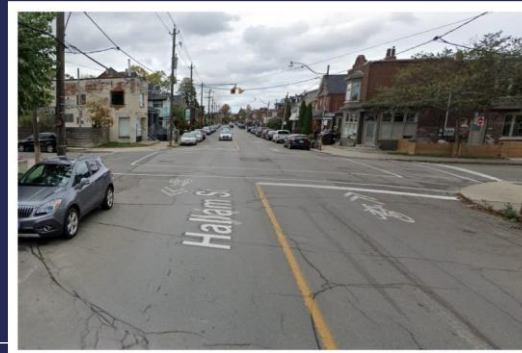
Example of Stop Bar (top photo)
